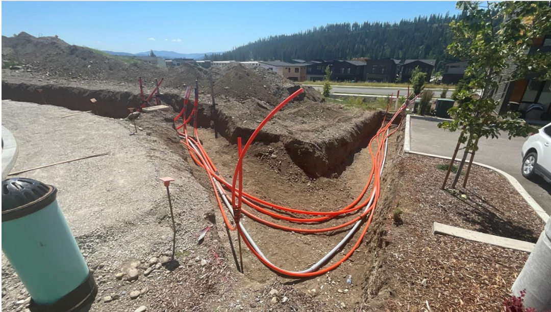
Photo of dry utility infrastructure installation on the project site.
