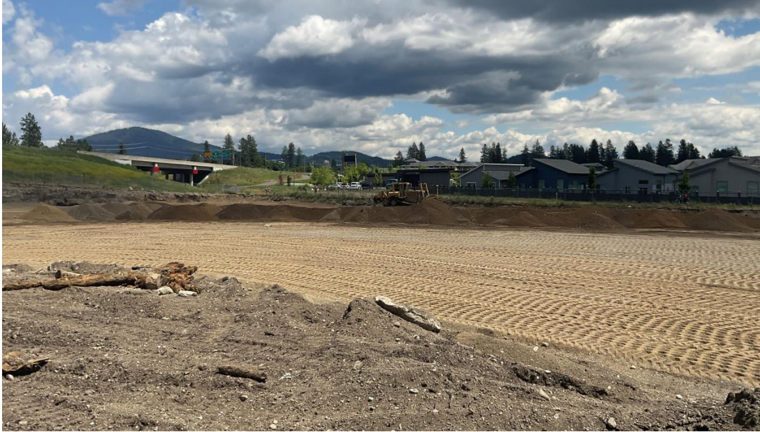
Photo of Atlas Road structural fill material placement on Atlas Project Phase 3 site.
