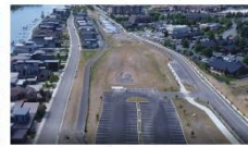
Lacrosse Roadway Extension - investment $1,782,000
