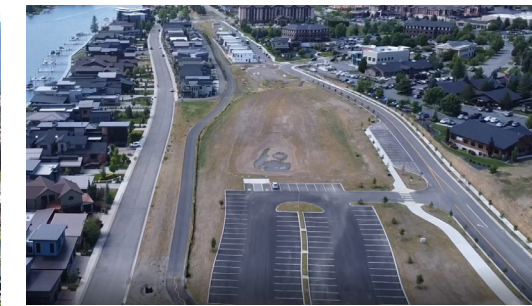
Lacrosse Roadway Extension - investment $1,782,000
