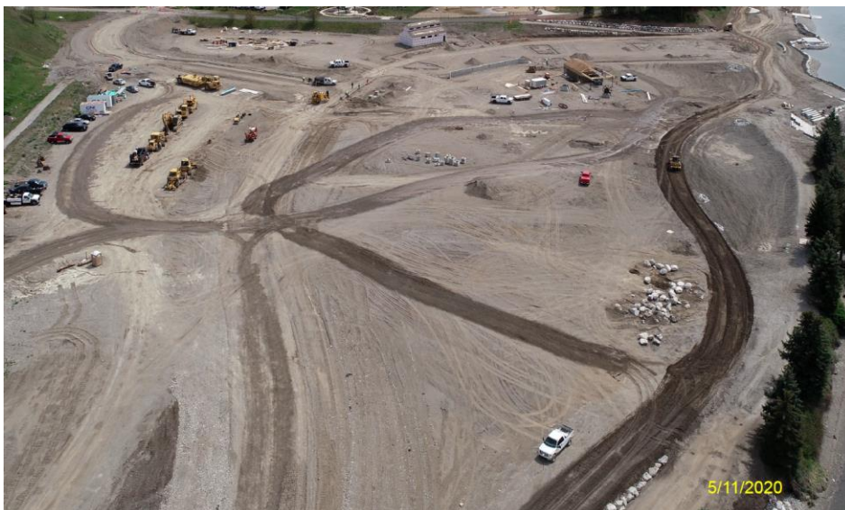
Project Site: Looking East
