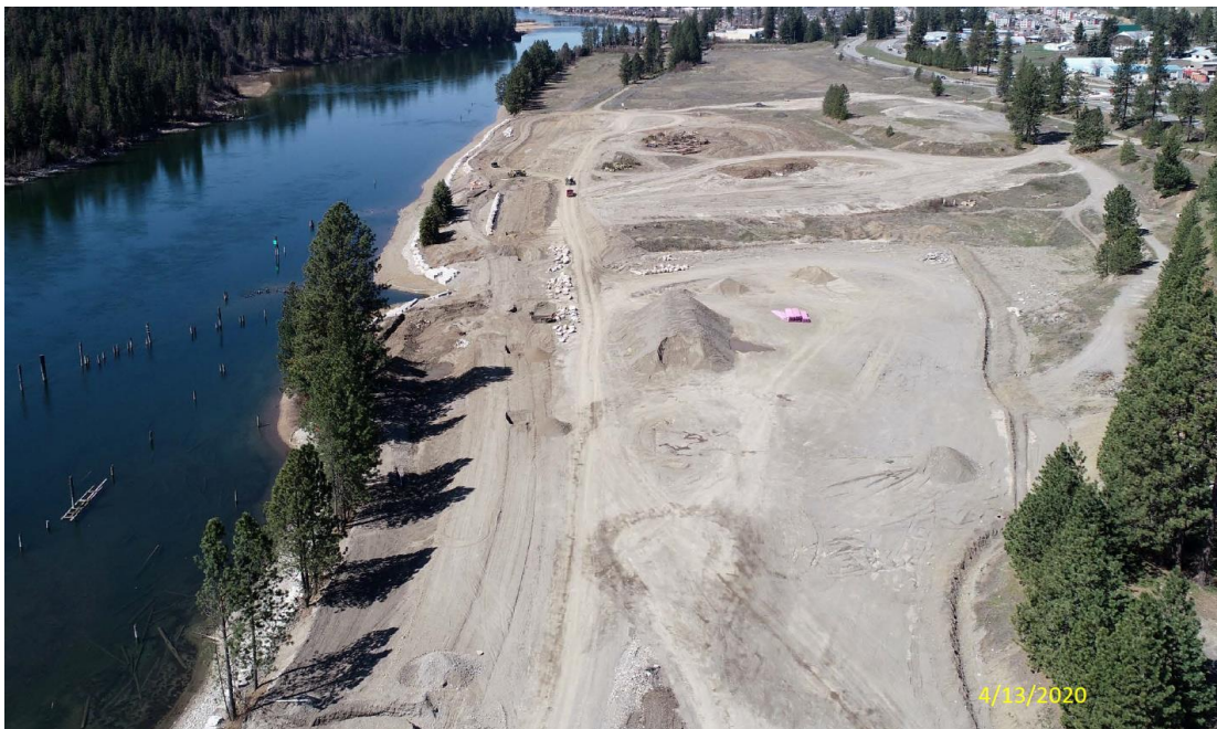
Project Site: Looking West.
