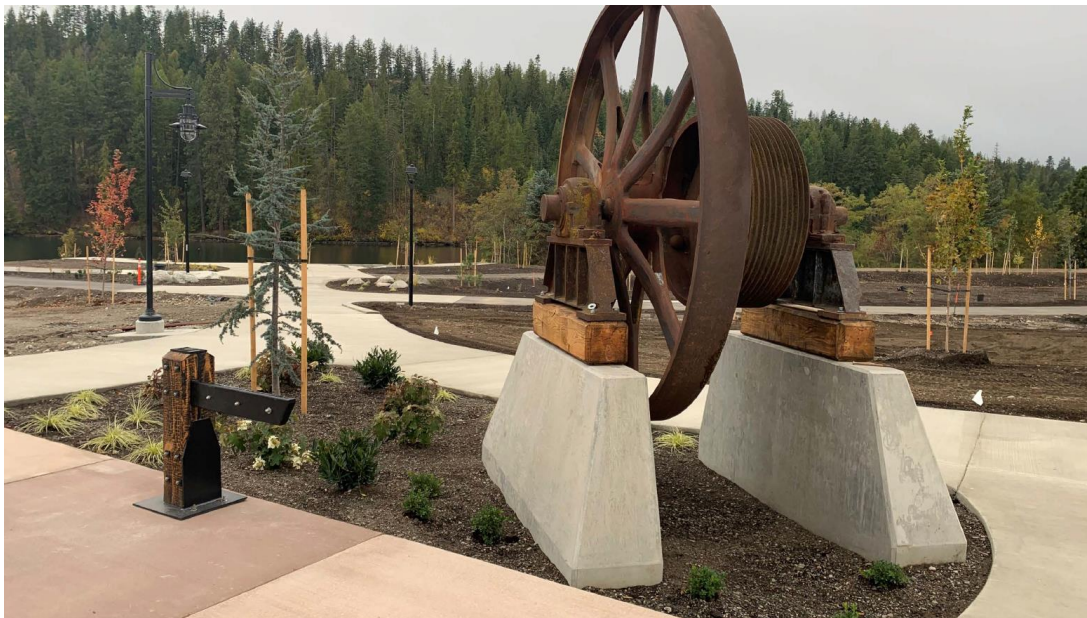
Project Site: Showing ongoing landscaping work and original mill flywheel.
