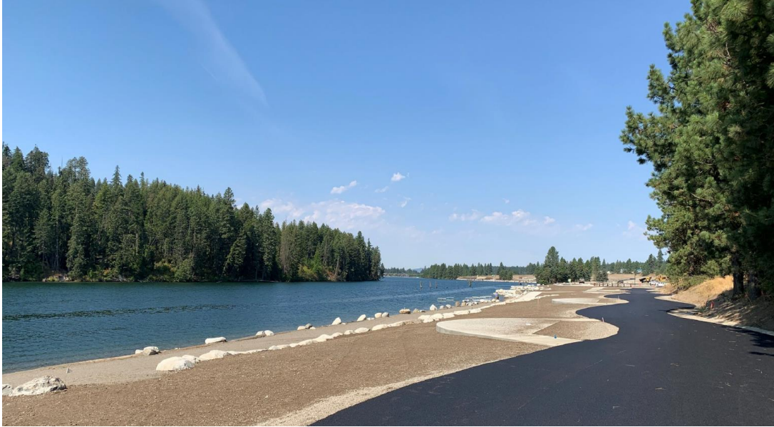
Project Site: Looking from East End to West
