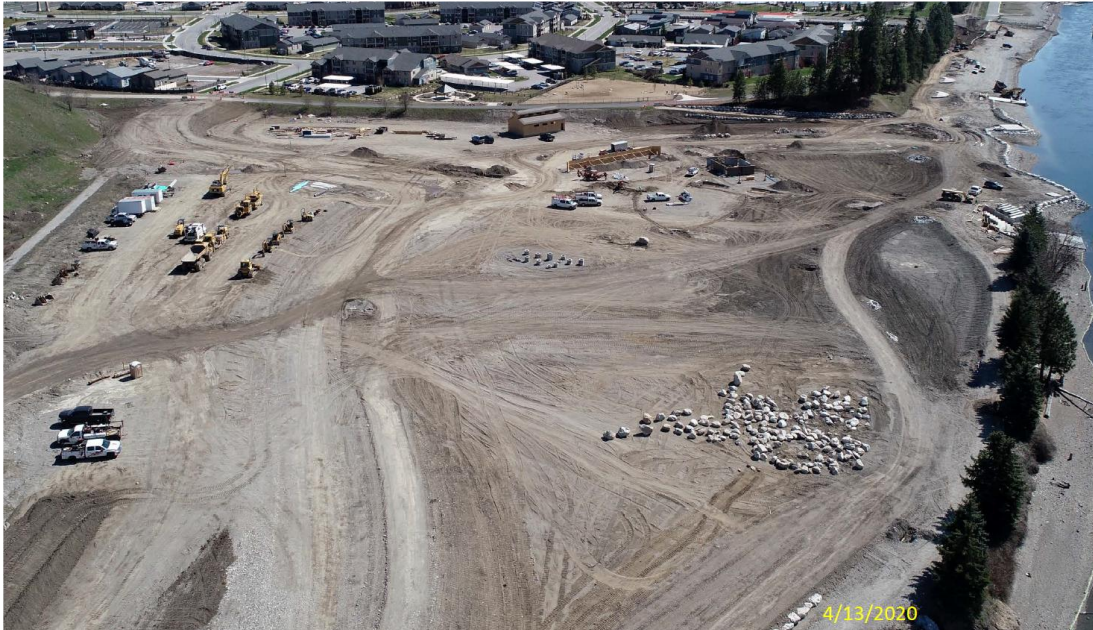
Project Site: Looking East
