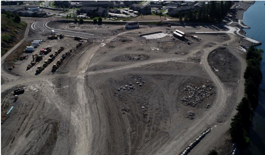
Project Site: Looking East
