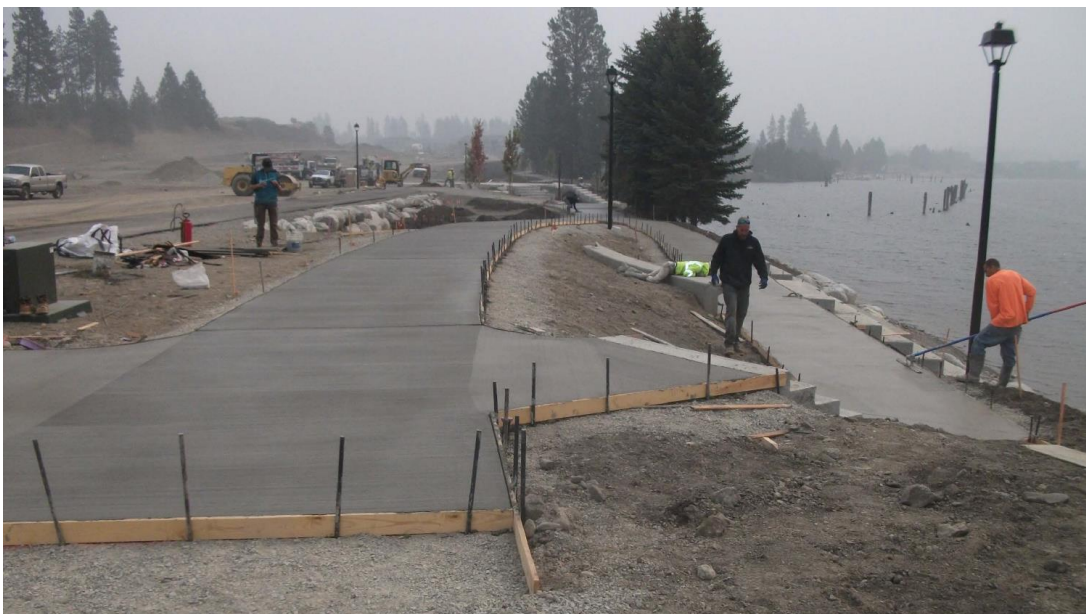
Project Site: Showing concrete flatwork located along the river's edge.
