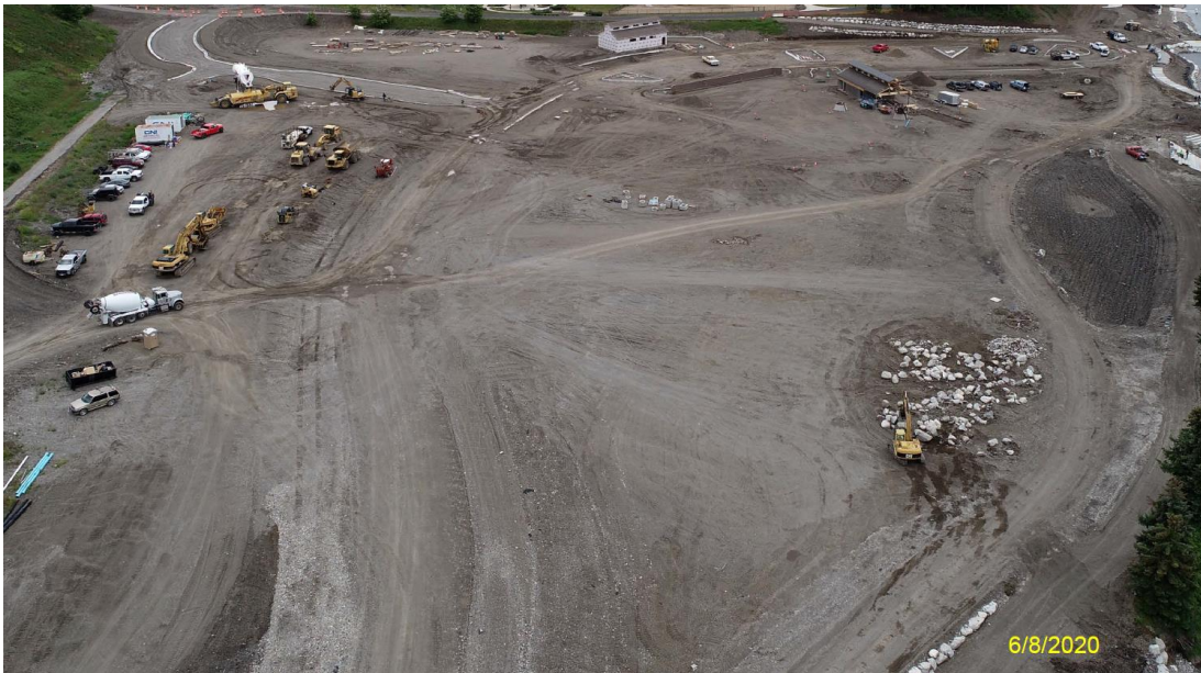
Project Site: Looking East
