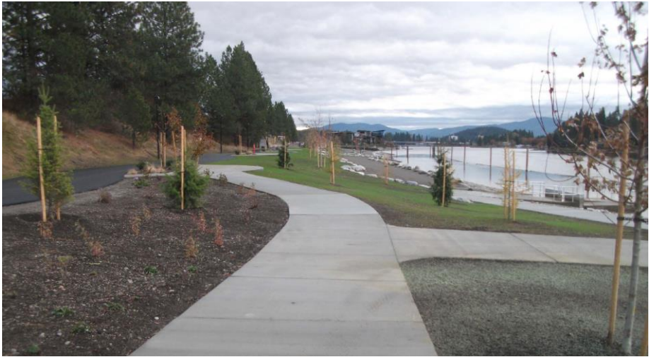
Project Site: View looking east from parking area.
