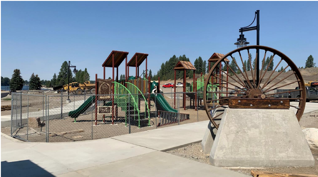
Playground Equipment Installation
