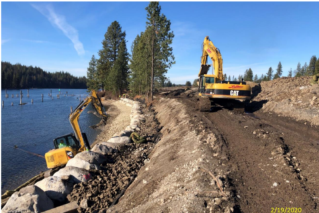
Project Area: Shoreline Stabilization Work
