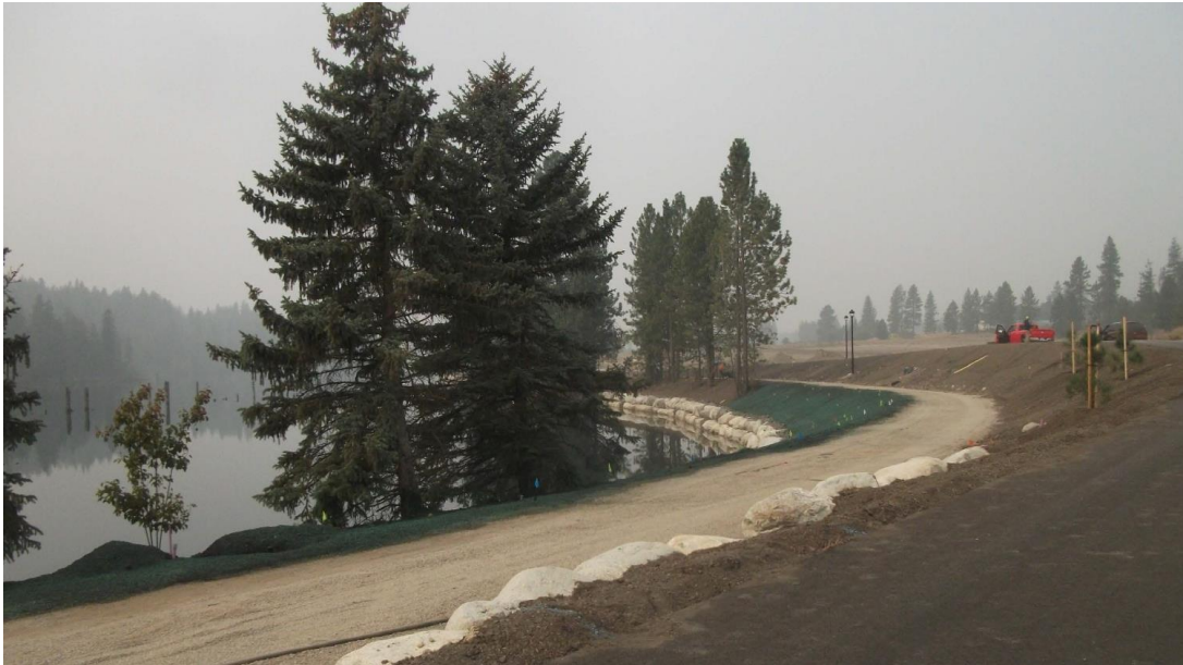
Project Site: Showing ongoing landscaping work.
