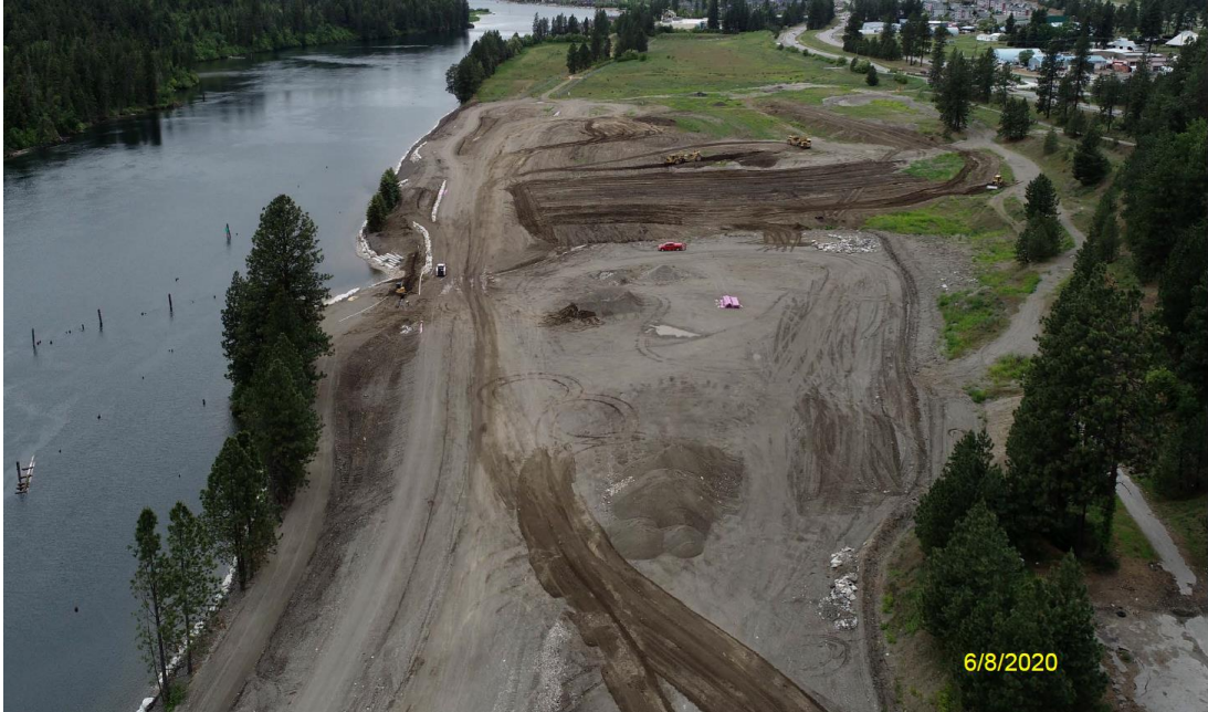
Project Site: Looking West.
