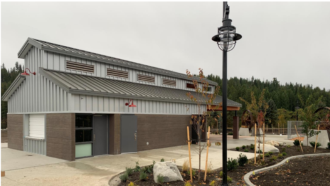
Project Site: Showing new restroom and picnic shelter building.
