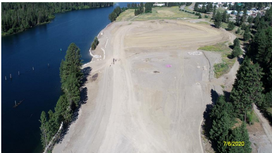
Project Site: Looking West.
