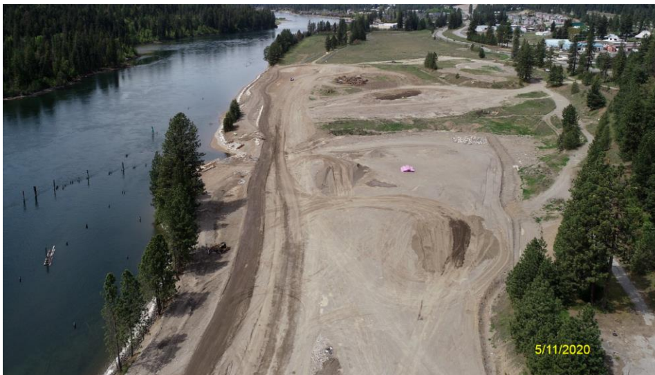
Project Site: Looking West.
