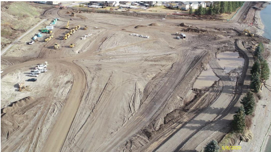
Waterfront project progress photo: looking east
